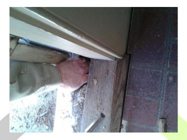
Rotted door threshold with more dry rot below in sub-floor and sill.
