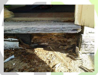
Door trim under threshold removed showing extensive dry rot in sill below
